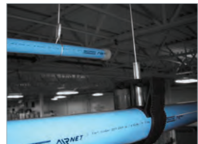
AIRnet piping installed with Gripper barrel fixing.
